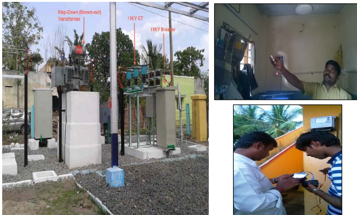
Fig. 4: The deployment in Madurthakam: Substation Deployment (left); UDPM and metering (bottom-right) and Household turning on DC devices (top-right)
